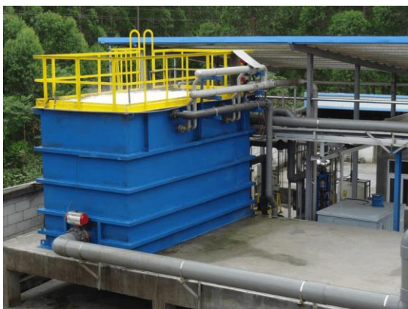
Photo 2: Membrane Bioreactor with submerged membranes of 60m 3 /hr capacity installed in China
