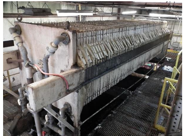
All recovered chrome containing floats are filtered to remove solids and fibres before storage in holding tanks for reuse.
