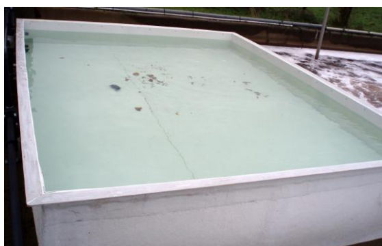
Picture: 2: Holding Tank with Nanofiltration permeate for water recycling.
